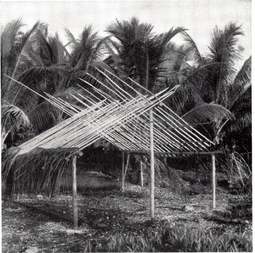
Fig. 20. House under construction. Lavanggu.
